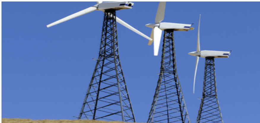
Figure 3.13 Lattice Tower
